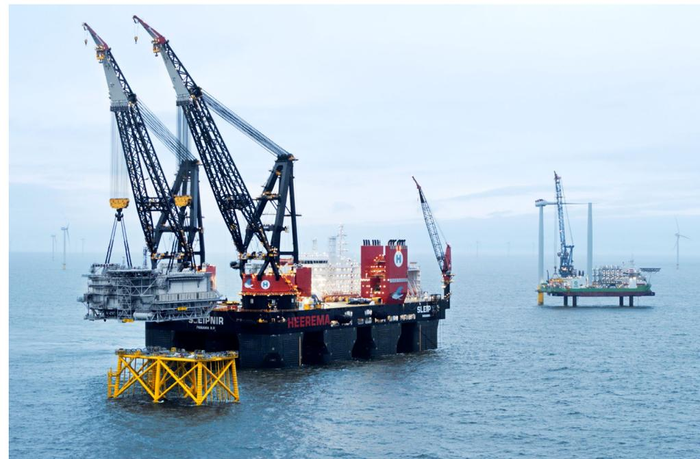
↑ Installation of the offshore substation at Hornsea 2, 89 km off the east coast of England.
